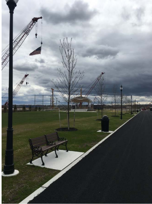
Recently completed Copper Works Park and Amphitheater with cranes from the NJ Transit Raritan River Bridge replacement project in the background.
